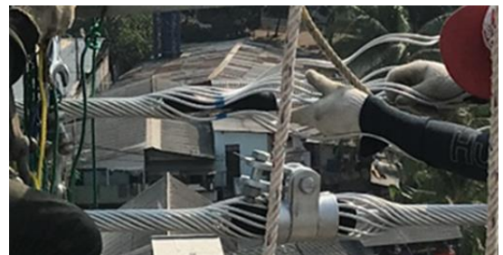
Installation of Armor rod and suspension clamp
