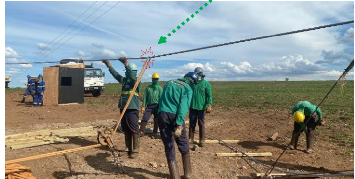
Use Hold-down \ Let-up block to avoid sharp bending
