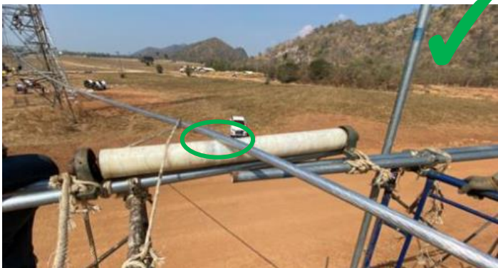
Roller should be used when pulling the conductor across obstacles
