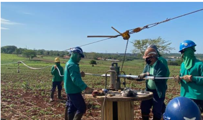
Installation of midspan joint on the ground
