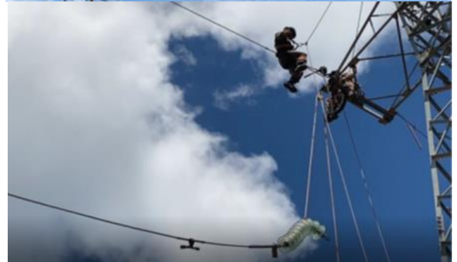
Installation of Deadend clamp on the ground
