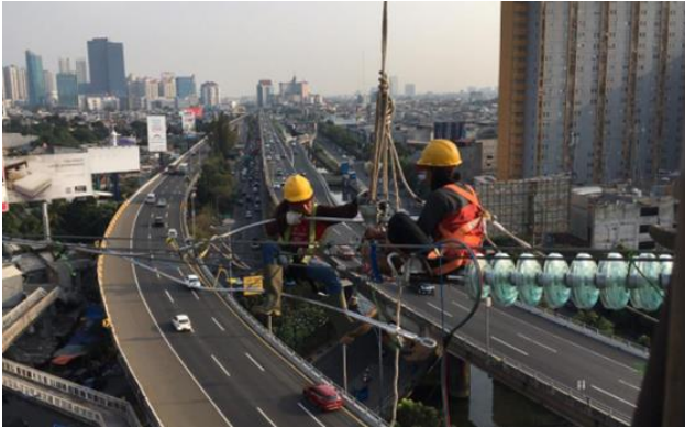
Installation of Deadend clamp on the tower
